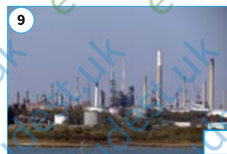
Fawley Refinery, Southampton Water
